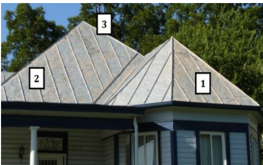
Historic standing-seam metal roof
